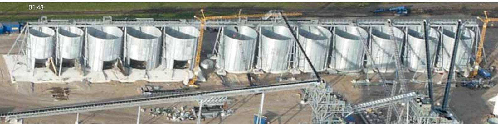
For gravel and ore treatment plants **silos** made of Hamco prefabricated steel parts have proven themselves. The positioning of the silos of a battery provides the storage of separated grain sizes without having long transports but with the full availability of the stored materials. (B1.43)
