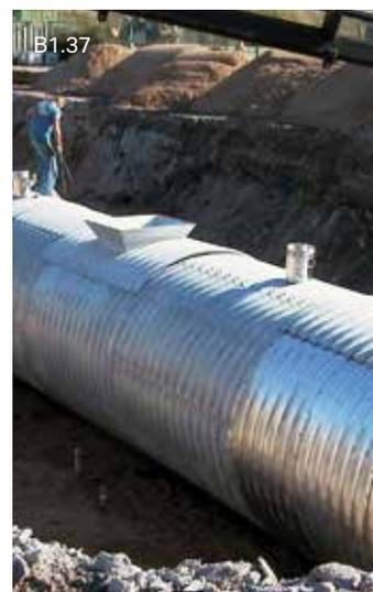
**Conveyor belt tunnel** made of Hamco corrugated steel parts have proven themselves below stock piles depending on the diameter up to 40 m height.
