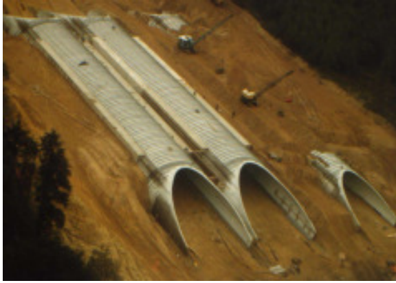
Picture 3: Greenbridge national park WoesteHoeve (NL) during construction
