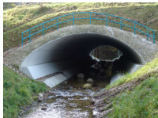
Picture 4: Completed corrugated steel pipes
